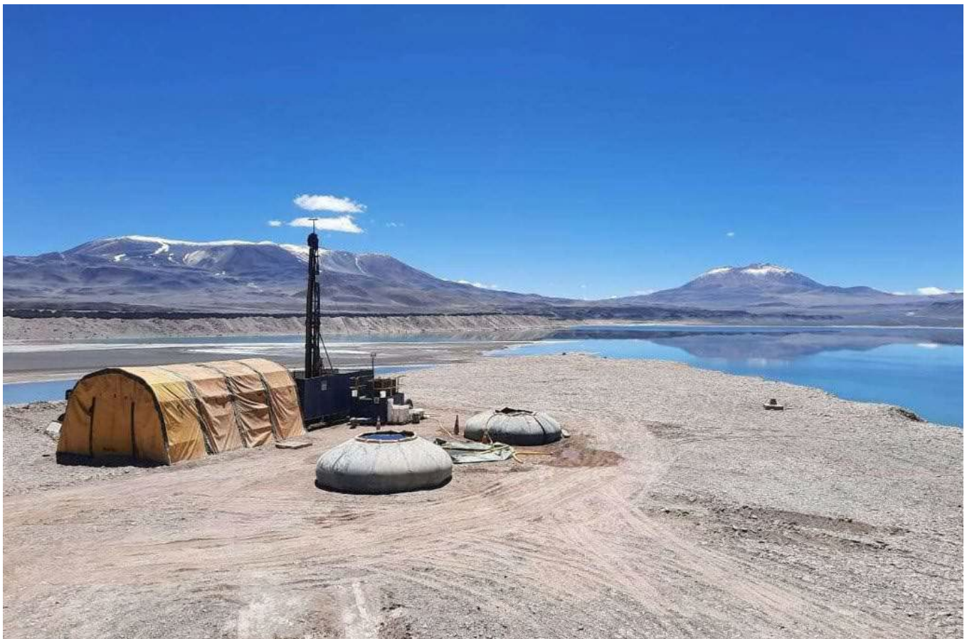
Figure 2: View from drill site (LV01) over Laguna Verde
